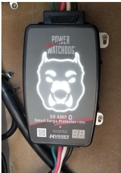
50 Amp Hughes Watchdog w/EPO (Emergency Power Off)
