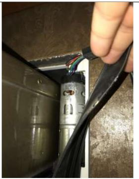
10. Get your new motor. Because your old motor was turned to a specific point when you took it out, you may need to manually turn the motor gear on the bottom so the new motor will "fall" into place. You will need a wrench and some strength to do this.
